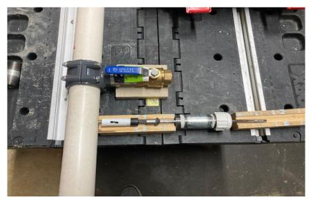
The hole saw is retracted into the 1" galvanized pipe nipple and then screwed onto the outlet of the ball valve.
