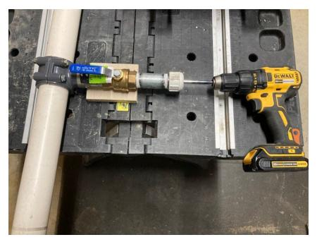
With the ball valve fully open, the hole saw is extended until it makes contact with the wall of the water distribution main. The drill powers the hole saw to provide a ¾" hole (tap in) in the wall of the pipe. The assembly is then retracted back through the open ball valve into the galvanized pipe nipple. The ball valve can then be closed isolating the water
