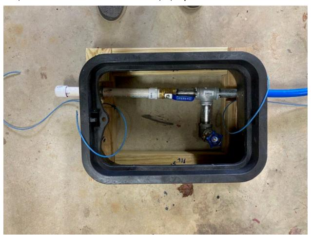
The above installation provides the property owner contractor a connection for temporary water service during construction. The hose bib connection can also be used for purging of the water distribution main and venting air during system maintenance.
