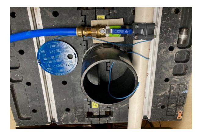
The above installation allows the tapping of the water distribution main under pressure. See Sec. 4 for complete construction detail and materials.
